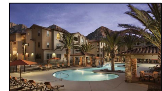
LUXURY APARTMENTS: VILLAS AT SAN DORADO
