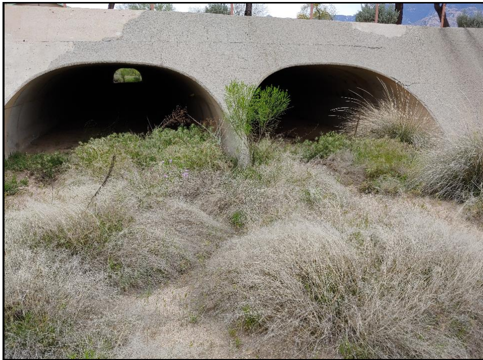
PHOTOGRAPH 22 Southern Culvert Facing North from Mitigation Area Towards Study Area
