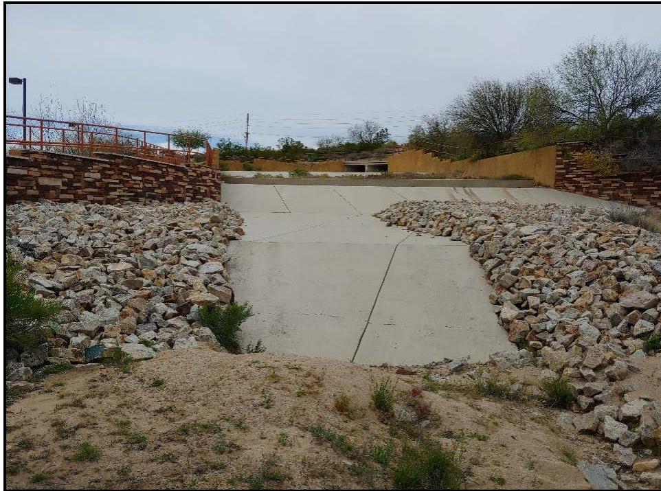
PHOTOGRAPH 23 Northern Terraced Drainage Feature, South of Tangerine Road
